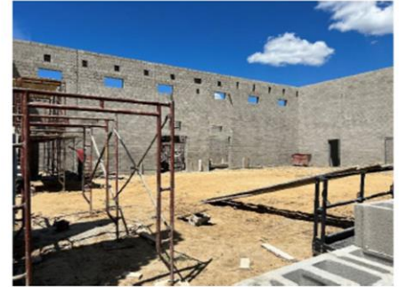
Block walls going up at addition
